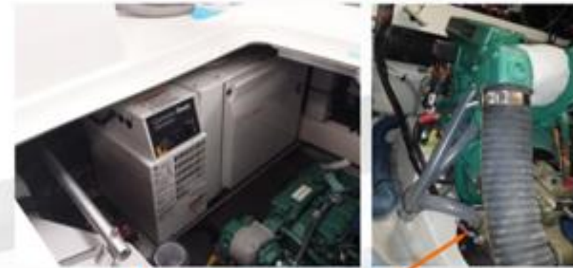
Seawater intake valve
